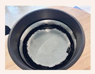
Open-top trough fitted with a watertight liner that extends 150 mm up from the base.
